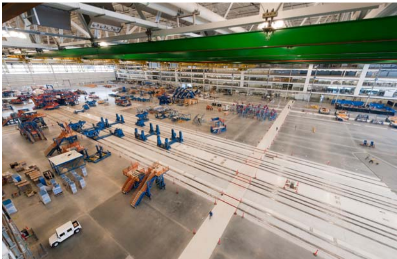
Boeing South Carolina 787 Final Assembly and Delivery Building North Charleston, South Carolina
